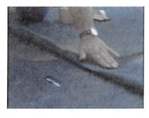
**Step 4**- Tack-back the overlap of the top PondGard panel using QuickPrime™ Plus Primer as an adhesive.
