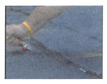
**Step 11**- Using a hand or stand-up roller; roll the seam longitudinally and across the seam in overlapping sections to mate the seam together.
