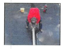
**Step 7**- Adhere the 3.00" (7.62 cm) QuickSeam Splice Tape to the primed surface of the bottom PondGard panel.
