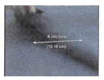
**Step 2**- Overlap the adjacent PondGard panels by a minimum of 4.00" (10.16 cm). Allow the PondGard panels to relax for 15 minutes.
