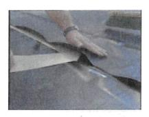
**Step 9**- Expose 0.25" to 0.125" (0.64 cm to 0.32 cm) of the tape outside the overlap. Remove the release paper and allow the top PondGard panel to fall across the tape while pulling the release paper away at a 45° angle.
