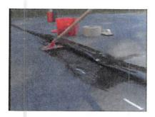
**Step 5**- Using a scrubber pad and holder; apply the QuickPrime Plus Primer to the bottom surface of the top PondGard panel and the top surface edge of the bottom PondGard panel.
